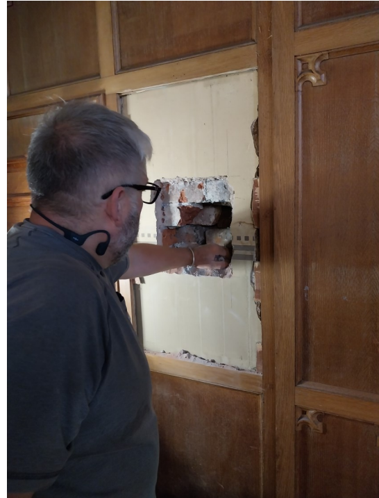
Lee cuts out the hole for the safe
