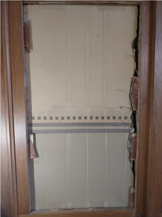
The wall panel removed revealing the 1930's colour scheme
